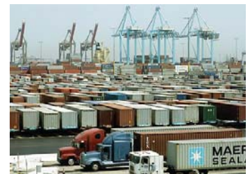
The Terminal Island Freeway is a heavily used route for trucks carrying cargo to and from the Ports of Los Angeles and Long Beach.
