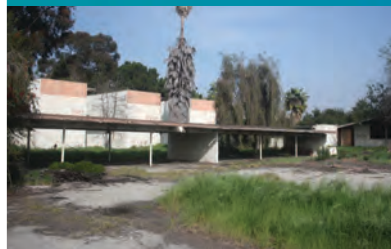
Anchor Place, before
